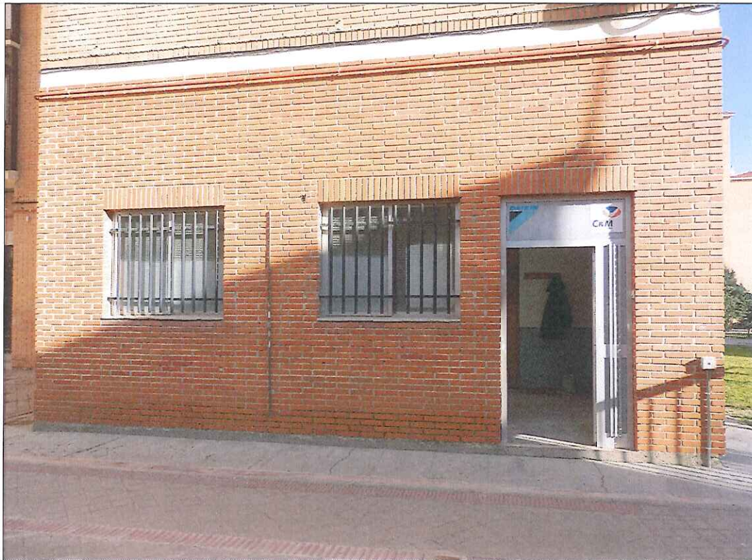
Detalle fachada principal
