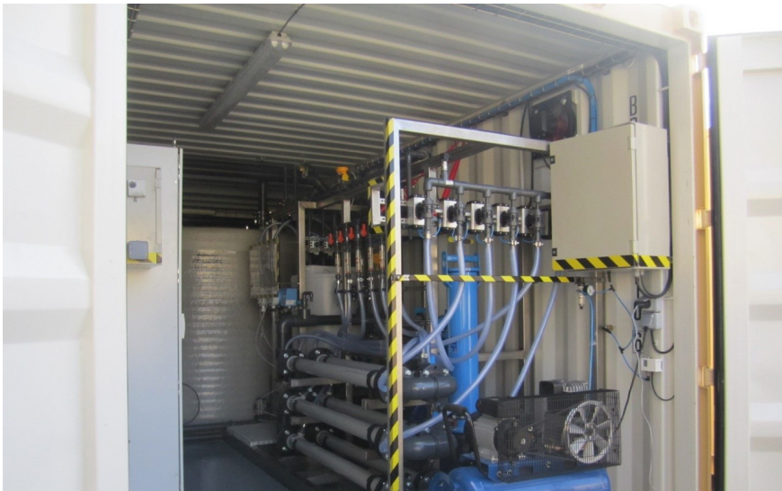
Figure 13. BRM biological treatment plant with external pressure membranes [online]. Source: https://www.protecmed.com/wp-content/uploads/2017/03/Ejercito-I.jpg [Accessed on: 2026]
