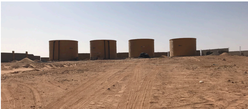
Figure 3. Water tanks in the Sahrawi refugee camps in Tindouf (Algeria). Own image
