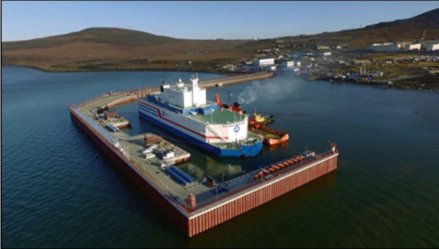
Figure 9: Floating nuclear power plant at Pevek
