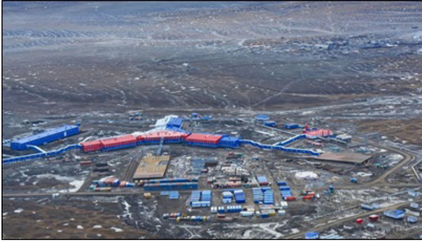
Figure 8. Severny Klever Base in Kotelnny, Sibir Islands
